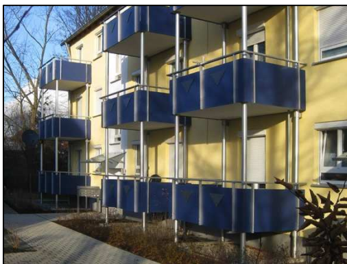
Figure 2. A stand-alone balcony (on the left) and a steel structure (on the right).
